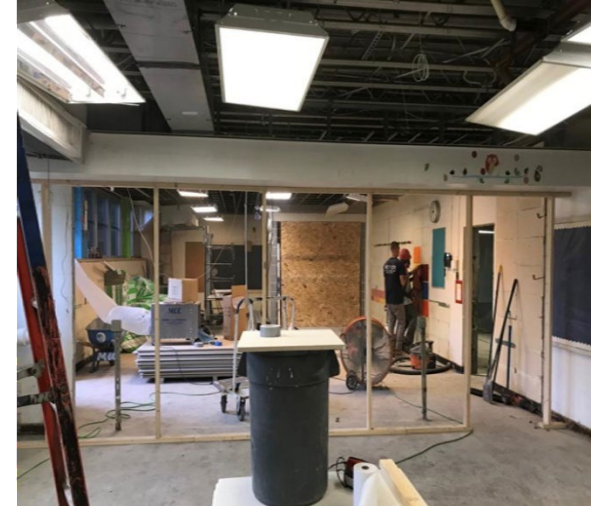
Demolition of Evans art and faculty rooms
